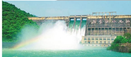
Excellent Repairing Project in Xinfeng River Hydroelectricity Power Station by using YDS-1
